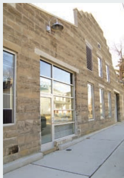
Maintenance and Training Facility
